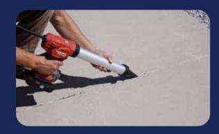
**2. Apply the Caulk** Using a caulk gun, a steady bead of caulk is inserted into and along the crack.
