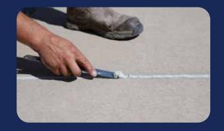
**3. Remove Excess** Excess caulk is removed with a putty knife to ensure a smooth surface.
