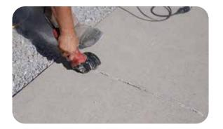
**1. Site Preparation** The existing mortar is removed using a saw, and the application area is thoroughly cleaned out.
