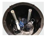
**Sump Systems** Once drained, a sump pump is needed to push water up and out of your basement through the discharge hose. To handle even the most extreme situations, we offer the S1 Single, S2 Double (with battery backup), and Super S3 Triple (with battery back-up + a 2nd standard pump).
