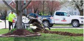
The trench is either dug by hand using a tile spade to remove the sod and excavate the trench, or a walk behind trencher is used to cut through the soil and create a smooth, even trench or installation.
