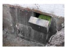
Install the Window Frame (if needed), then Window, and finally the Window Well itself.
