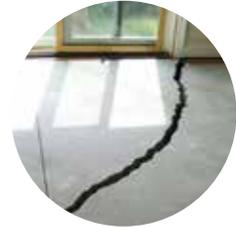
One major fallback to slab foundations is that they are constructed in the active soil zone, which is affected the most from seasonal wetting and drying.
