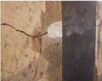
In addition to our high strength Polyurethane to fill the existing void, Helitech utilizes the CarbonBond Structural System as a reinforcement of concrete and block basement walls. High tensile strength Carbon Fiber sheets are often installed over crack injection work to stop any further movement. With Carbon Fiber materials stronger than steel, CarbonBond bridges the forces to fix the crack.
